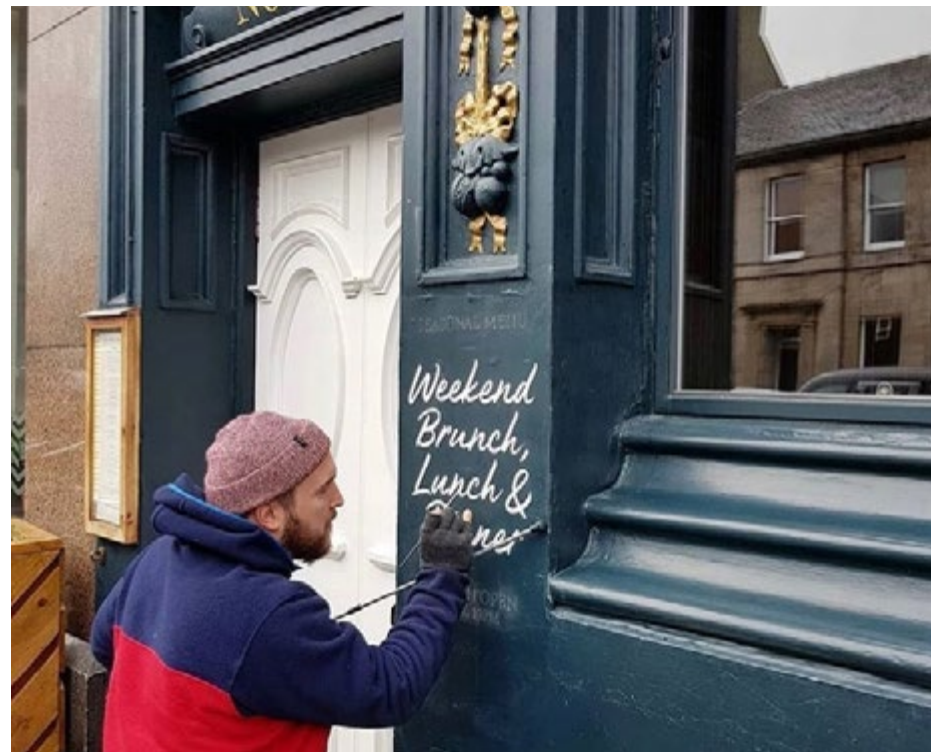
4.17 Hand painted pilaster signage (Thomas Paints).
