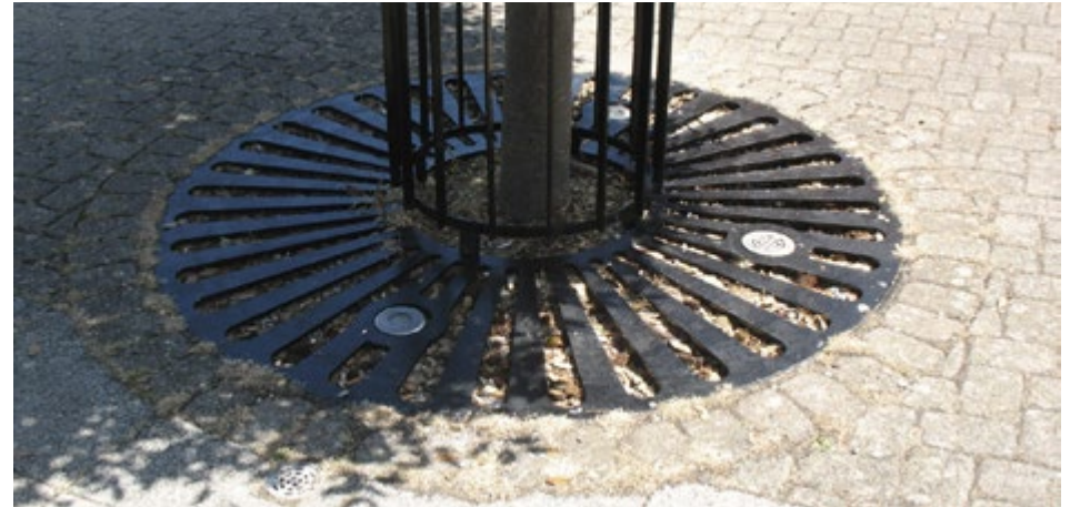
6.35 Paving should be neatly finished around tree grilles (©GreenBlueUrban)
