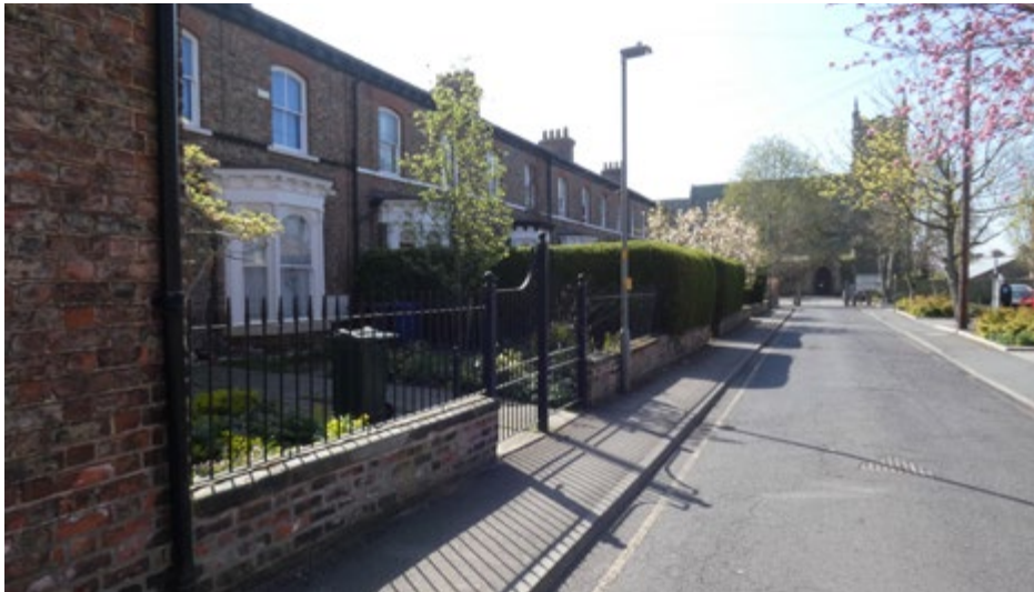
2.16 Dwarf brick wall with railings (Insall)
