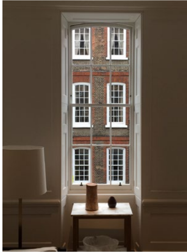
4.10 Refurbished windows and new shutters (Insalls)
