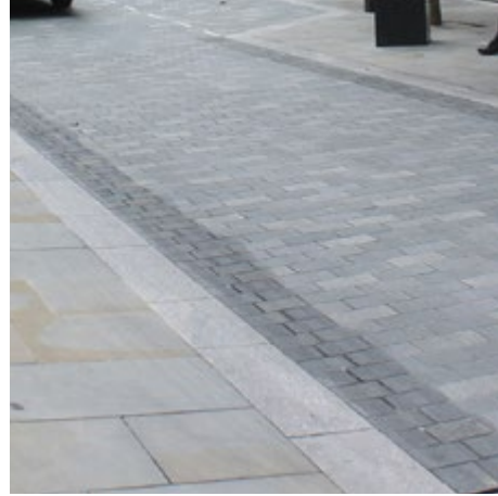
6.2 Flush kerbs help promote the sense of a 'shared space' on Bourdon Place, London
