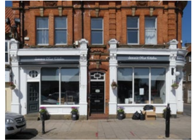
3.5 Late-Victorian shopfront on Micklegate (Insal)
