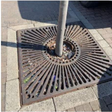
6.40 Cast iron tree grille on Micklegate
