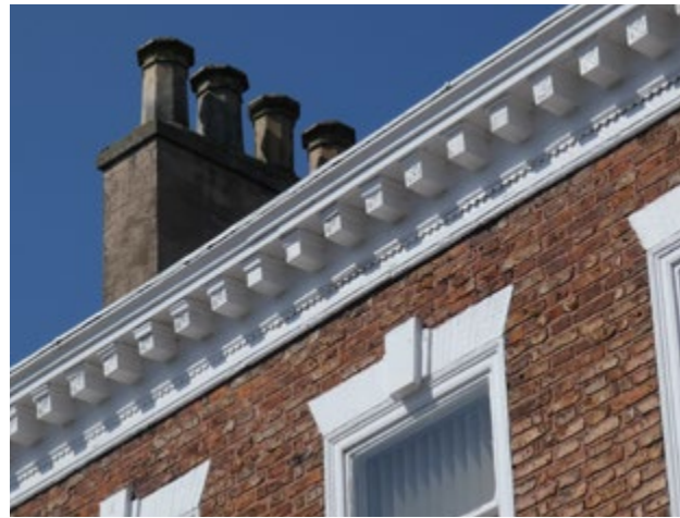
4.4 Well-maintained timber eaves cornice (Insall)
