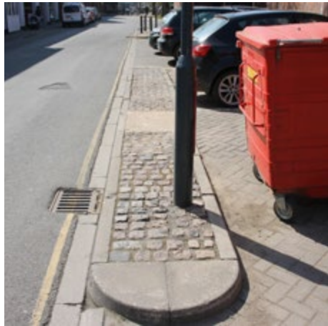
6.5 Channel edging to road surface with small unit setts used as fill, on James Street
