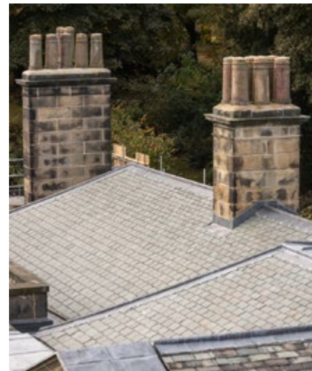
5.2 Newly laid natural slate roof (Insalls).
