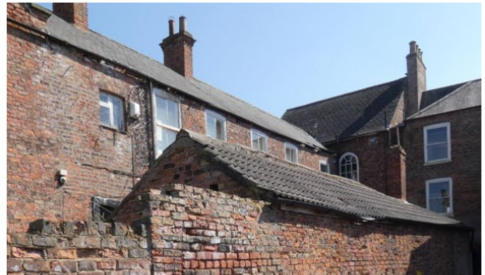
2.10 Rooflines of rear extensions at 90 degrees to the street frontage (Inshall)
