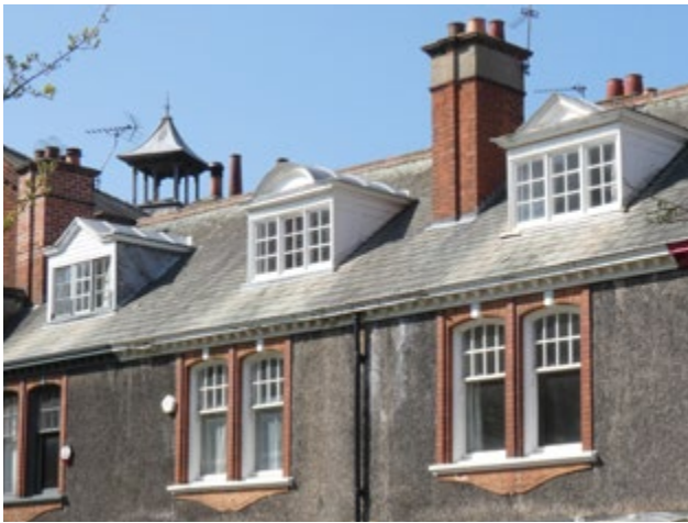
4.3 Slated roof with dormers to Edwardian property close to the Abbey (Insall)
