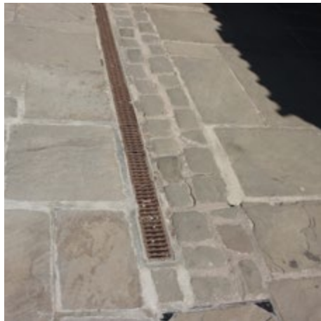
6.13 Integrated drainage details
