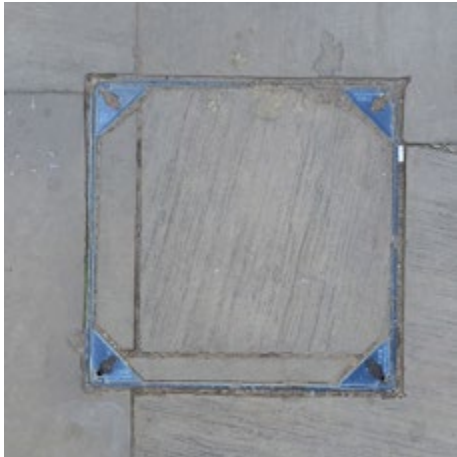
6.9 Neatly finished recessed service covers should be used where possible
