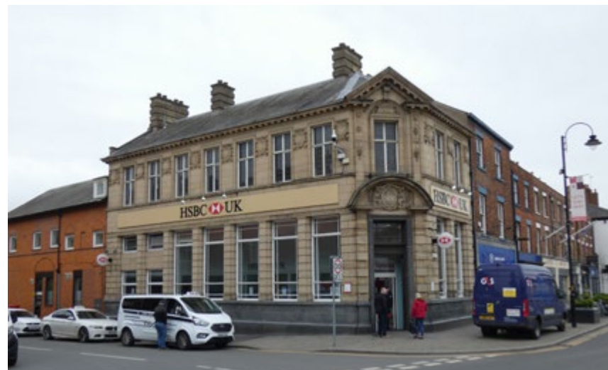
5.12 Bank at the corner of the Market Place and James Street (Inshall)
