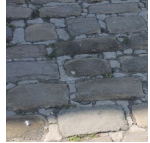
6.4 Historic paving should be retained where possible, on Micklegate
