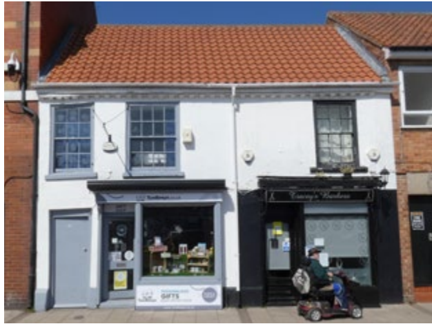
3.3 Mid-Victorian shopfront retaining awning fixings (Insal)
