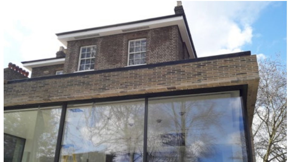
5.1 New extension with brick carefully matched to the historic main building (Insalls)
