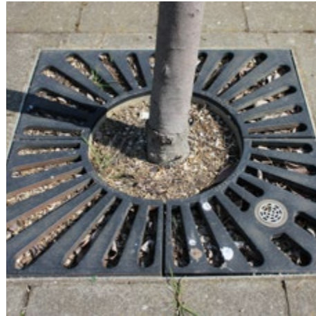
6.34 Tree grille finished in matt black, with aperture for fixing the inlet of an aeration/irrigation system on Riverside Gardens
