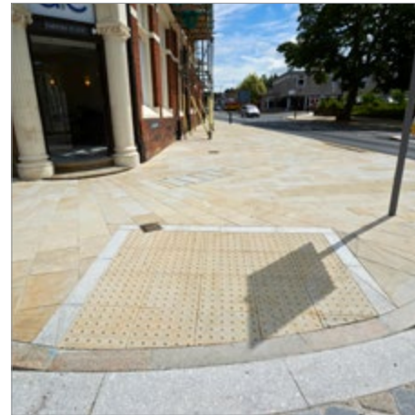
6.7 Tactile paving should be tooled from Yorkstone where possible (Image Source: Marshalls)
