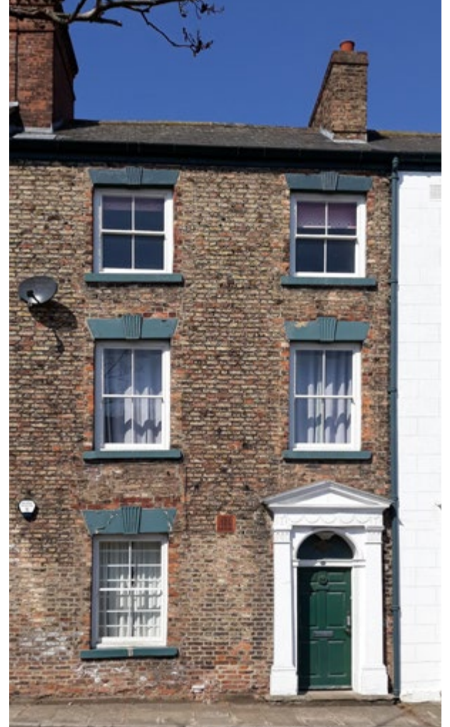
4.5 Colour-matched and neatly-arranged rainwater goods (Insall)
