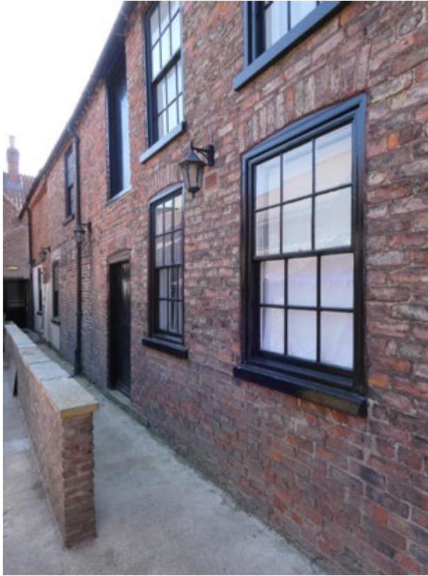
4.9 Combination of refurbished and replacement Georgian sashes (Insall)
